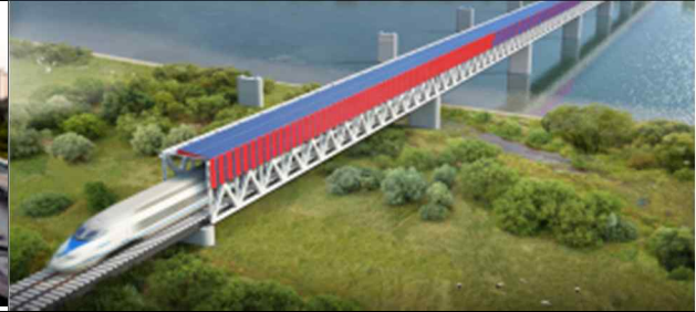
<Solar Power Facility on Imjingak Bridge near Dorasan Station>
